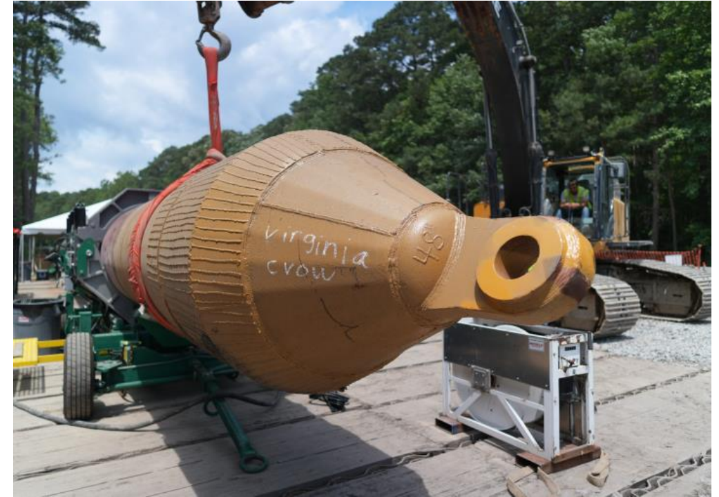
Horizontal directional drilling on the Coastal Virginia Offshore Wind project
