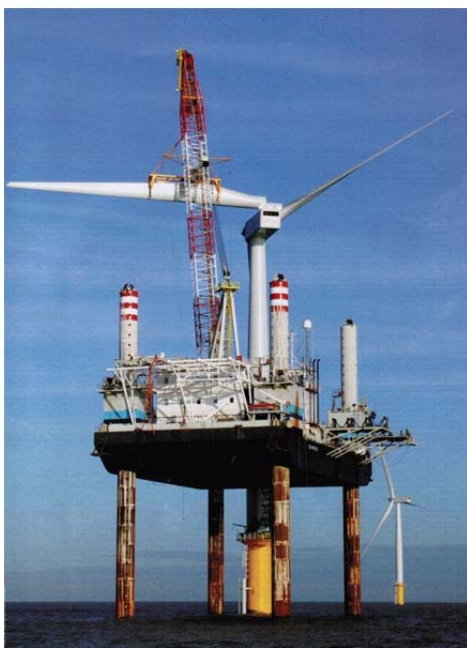
Figure 7. A large mast-mounted turbine being installed in the Irish Sea.
