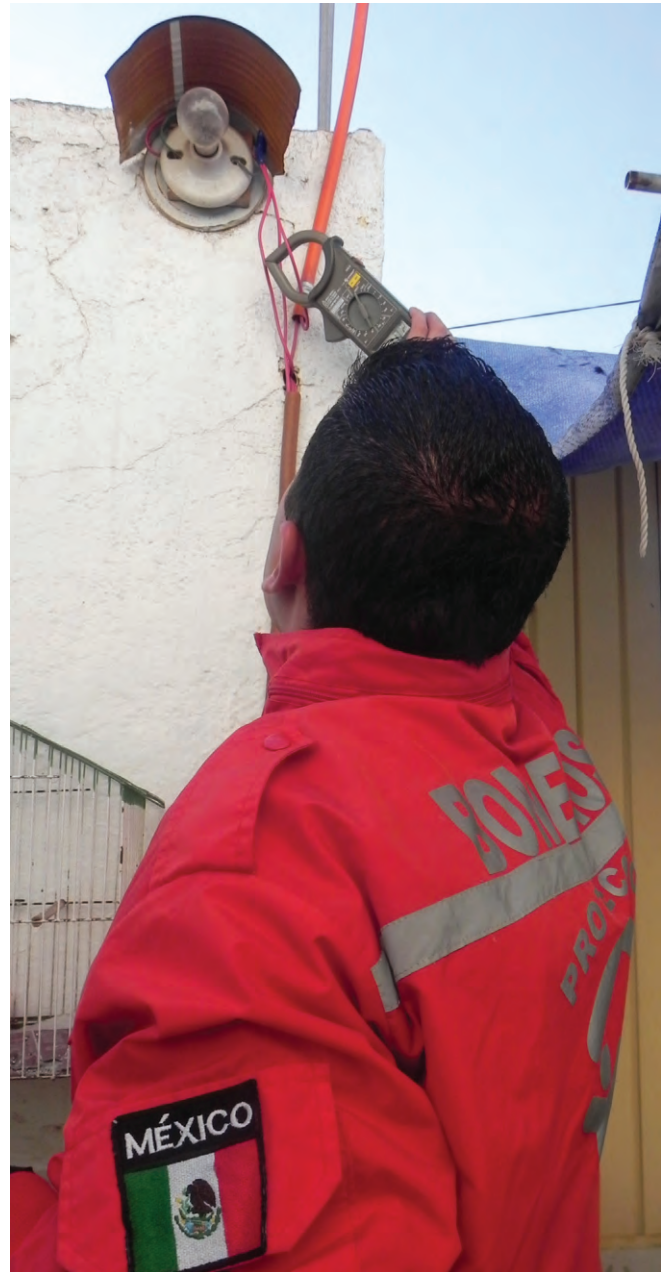
Figure 18 Inspecting the electrical installation in a house
